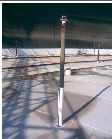
Figure 2: The deck leg of storage tank.
