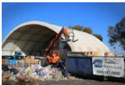
Figure 1: CleanWorld's anaerobic digester biorefinery which processes 40,000 tons of food waste annually for the production of biomethane for transportation applications.
