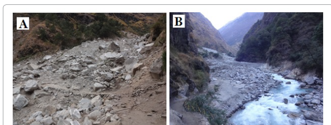
Figure 3: (a) Gully erosion in the old landslide mass on the left bank of Malpa Gad, (b) accumulated sediments along the Kali river banks in the area round Malpa.
