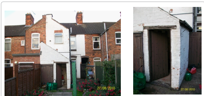
Figure 4: a) Rear elevation b) Existing outbuilding.
