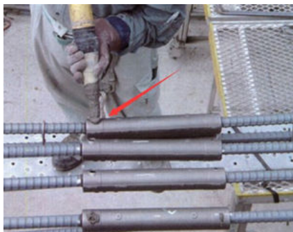
Figure 1a: Sleeve grouting connection.
