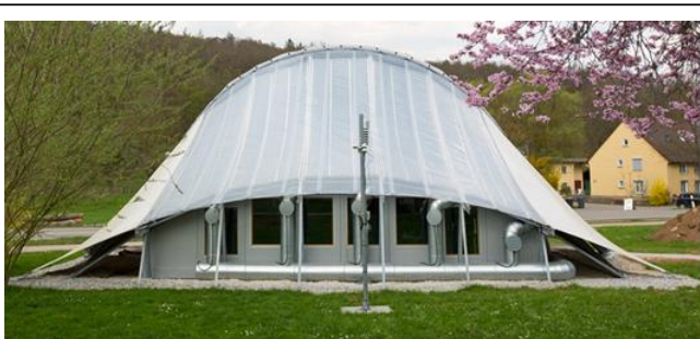
Figure 2: The polar bear pavilion, inspired by the solar thermal functions of the polar bear's fur.
