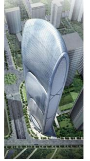
Figure 14: Zero-energy skyscraper «Pearl River Tower» [23] (spiral "wind vents" are visible on the right side of the house, solar panels are on the facade).
