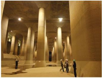
Figure 7: "Water pressure control bath" (size 178x77x18 meters).
