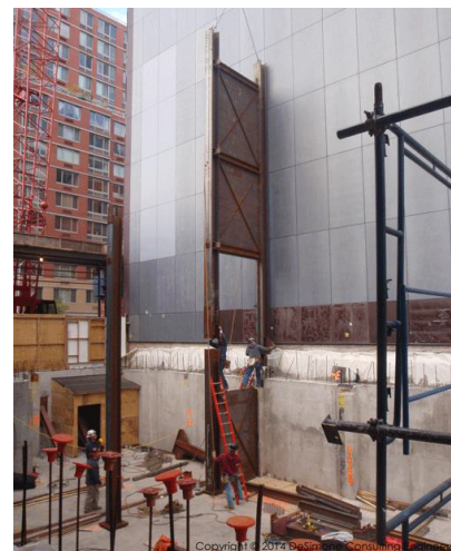
Figure 5: High Line 23 Steel Plate Shear Wall Installation (Copyright 2014 DeSimone Consulting Engineers).
