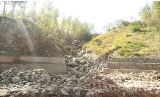
Figure 3: View of broken retaining wall due to landslide at Sanadi area.
