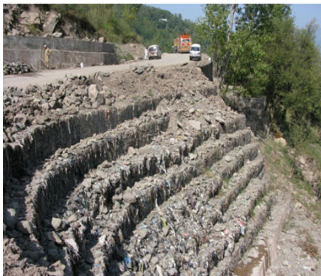
Figure 6: View of newly constructed retaining wall in Sanadi area.
