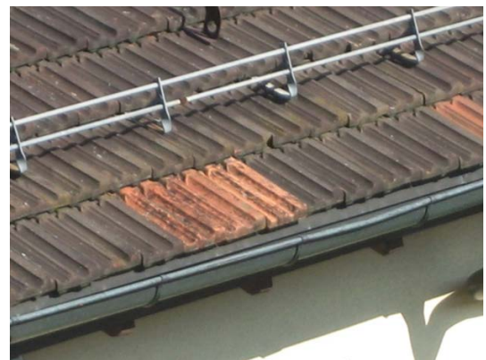
Figure 17: Roof with recently substituted bricks.
