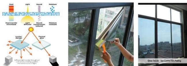
Figure 10: Sun Control film pasting over glasses.
