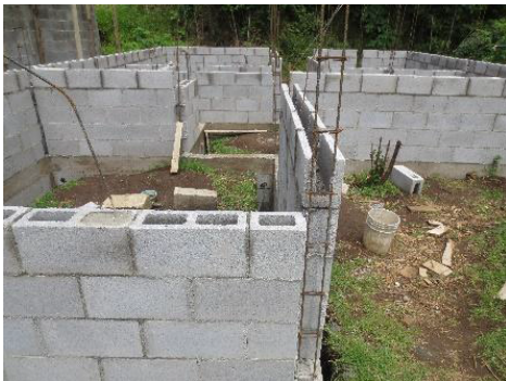
Figure 9: House under construction, cooperative Fe y Esperanza, Guatemala.
