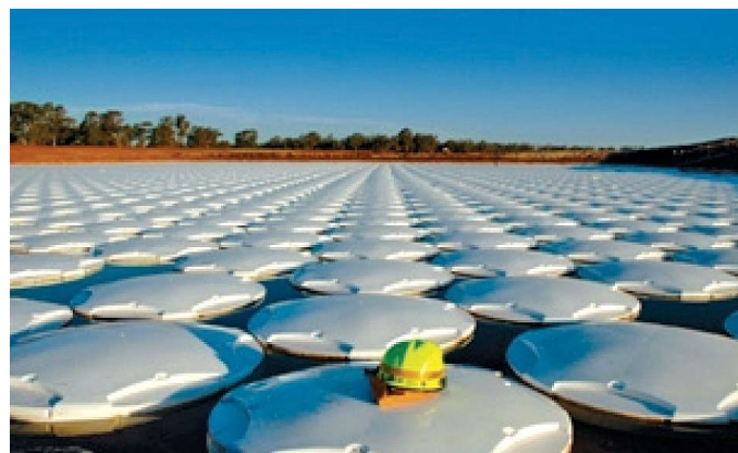
Figure 4: Untethered tiles on a mine reservoir at Parkes in Australia (Aquacap brand, 2010).
