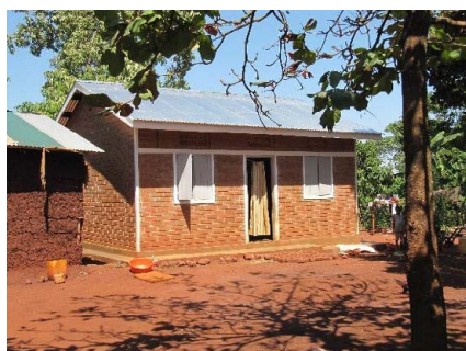
Figure 10: Basic house of CEB built in Uganda (Oskam v/f).
