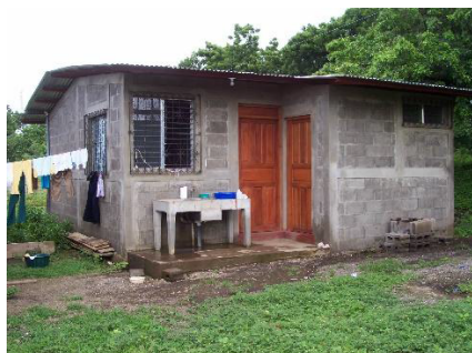
Figure 20: House built with hollow concrete blocks, Nicaragua.
