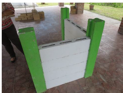
Figure 22: Prefabricated concrete panels by FUNDASAL in El Salvador.
