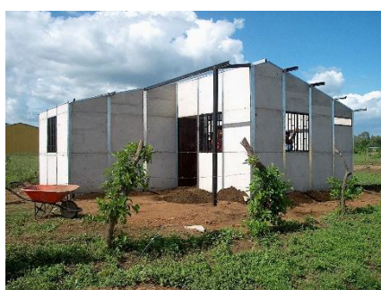
Figure 21: House with concrete panels within an aluminum framework, Nicaragua.
