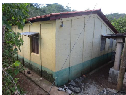
Figure 23: House with concrete panels in Piedras Rojas, El Salvador.
