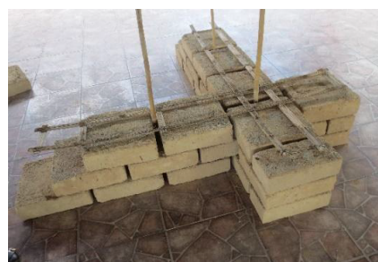
Figure 12: Corner solution for adobe walls with reinforcement.
