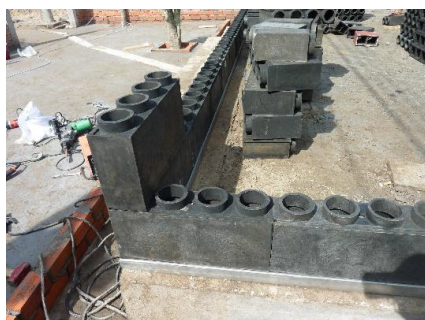
Figure 16: Construction of community house with RHPP in Vinh Thanh village, Vietnam.
