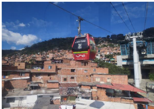
Figure 4: Cable car track in Medellin, Colombia.
