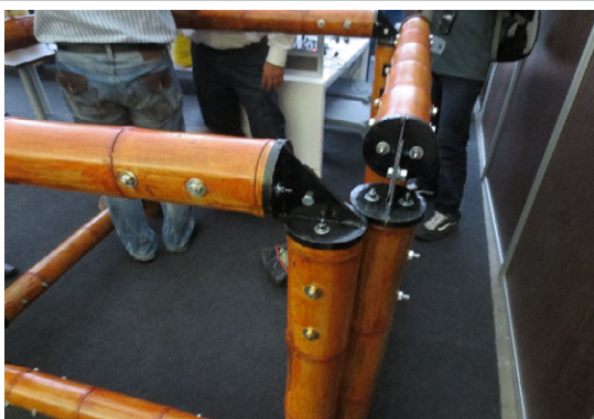
Figure 6: New bamboo corner joints suitable for housing.
