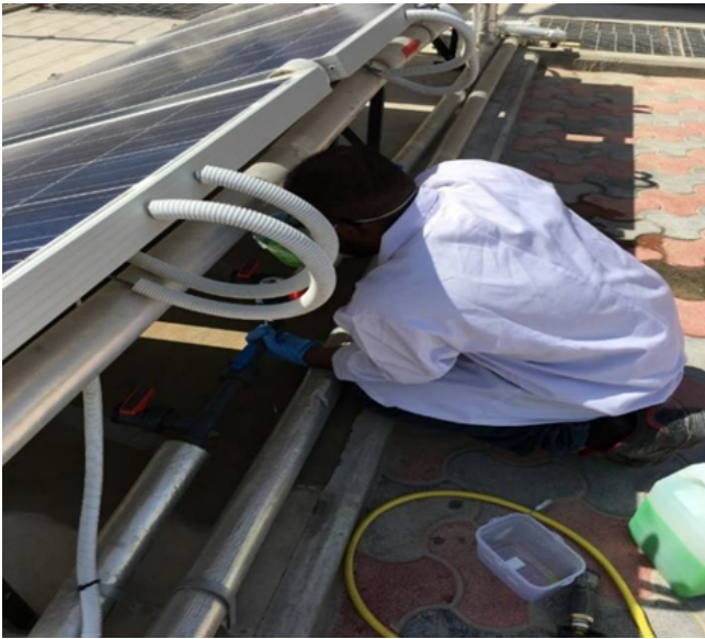
Figure 4: Insertion of Nanofluid in the PV/T closed hydronic circuit.
