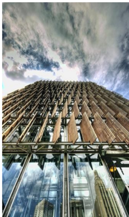
Figure 8: Council House 2 (CH2), main façade.
