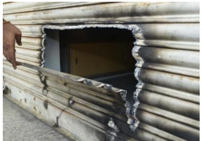
**Figure 1:** Shutter broken by gas cutter.
