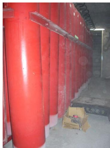
Figure 1: Liquid carbon dioxide steel cylinders in basement.
