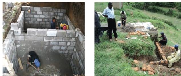
**Figure 5:** (a) On the left, the building process of the designed septic tank for a selected primary school of 150 students (b) on the right, the completed septic tank.
