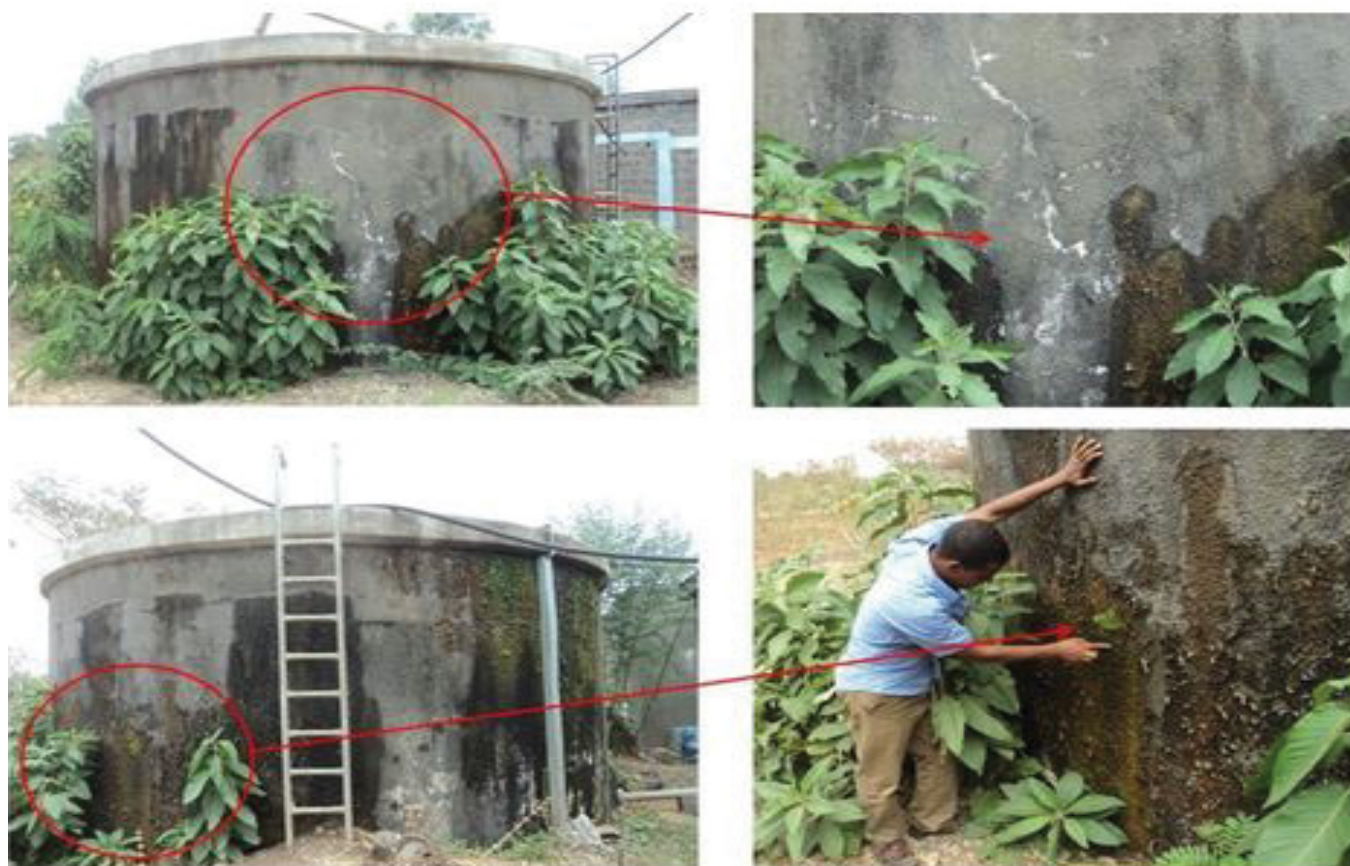
Figure 2: Surface deterioration of 15 years aged RC storage tank, Ethiopia (concrete made from Messobo OPC).
