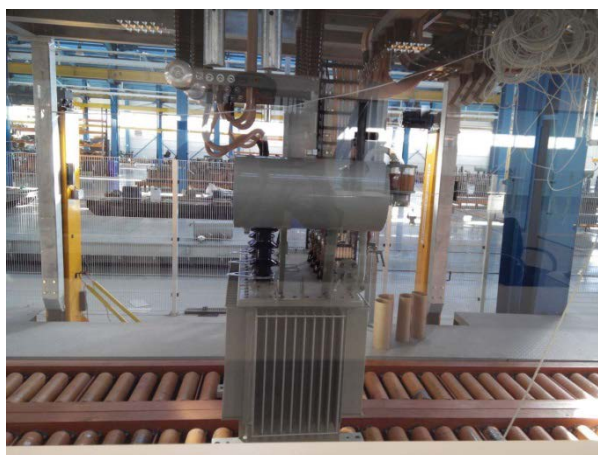
Figure 4: Transformer test object.
