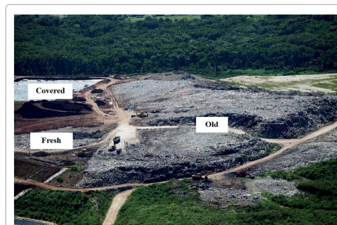
Figure 2: This figure shows the waste dome with these three parts: fresh, old and covered waste.
