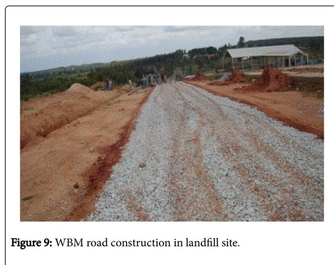
Figure 9: WBM road construction in landfill site.
