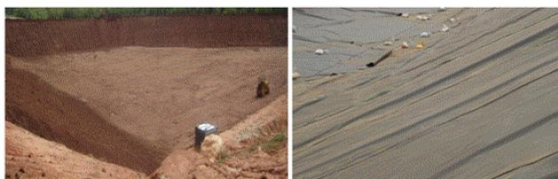
Figure 7: Liner system at base and side of landfill.
