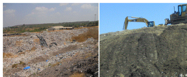
Figure 6: Typical construction procedures of soil cover.
