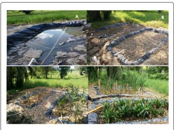
**Figure 1:** a) Fluid distribution system; b) Filtering bed used; c) Initial sowing of vegetable patterns; d) Vegetation adapted to the system.
