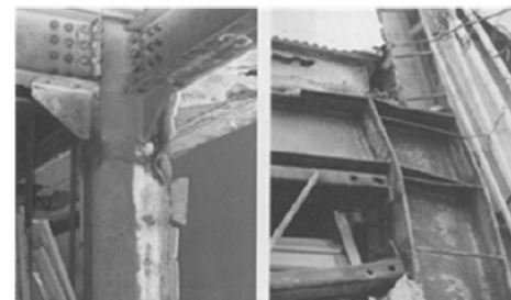
(a) Example of damaged steel frames (the Great Hanshin-Awaji Earthquake, Japan, 1995)
