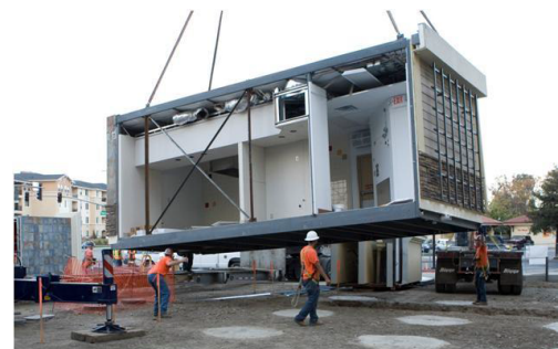
Figure 1: 'Module' being lifted by a crane.
