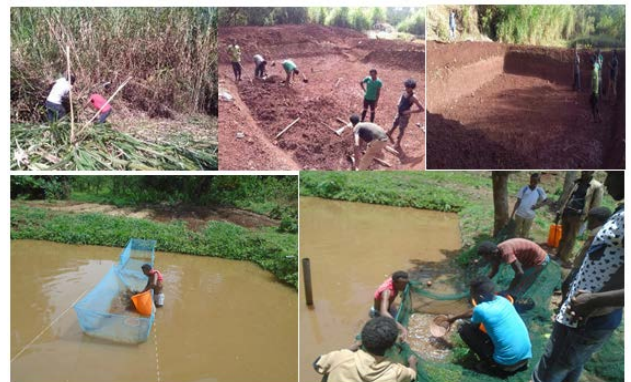
Figure 1: Site clearing and pond Construction at Wayu Tuka FTC, data collection from Hapa system and demonstration.
