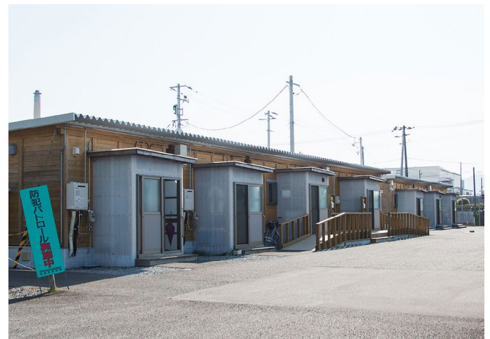
Figure 1: Various forms of temporary housing.
