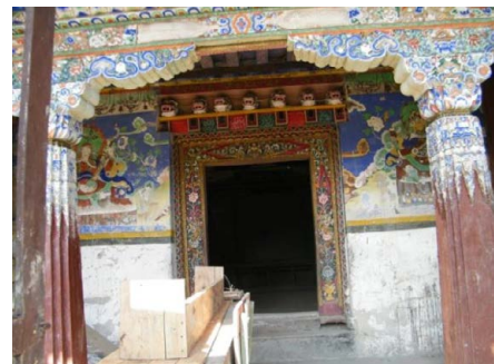
Figure 13: Timber Columns in front of Verandah.
