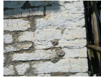
Figure 10: Rubble masonry.
