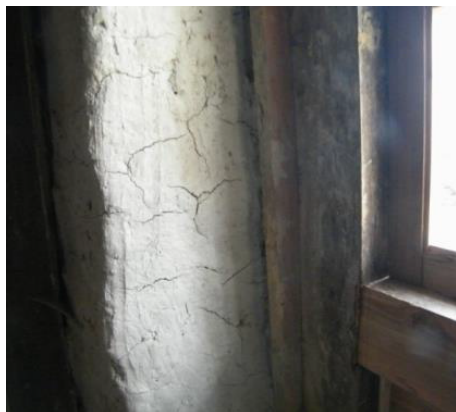
Figure 21: Plaster cracks.
