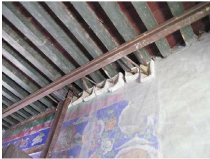
Figure 14: Wooden Rafter and Planks.
