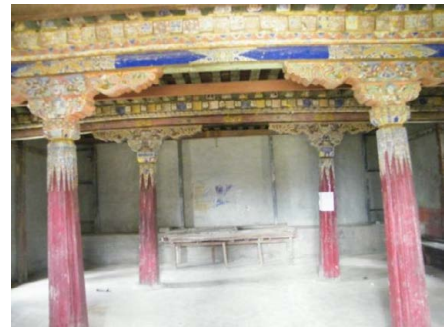
Figure 11: Wooden columns and beams inside the Hall.
