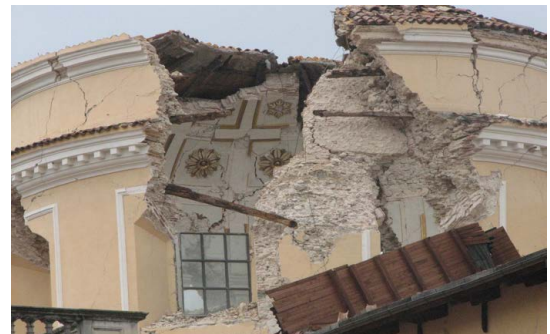
Figure 4: The destruction of the dome (the greatest destruction of the dome coincided with the direction of the seismic wave front) of the Catholic church in the town of Aquila in the province of Abruzzo in Italy, after the devastating earthquake in 2009.
