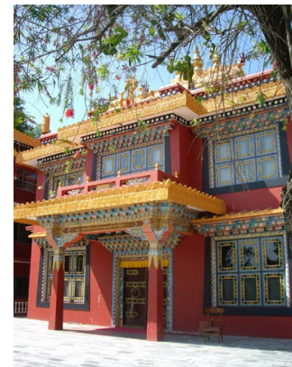
Figure 5: The Buddhist temple in the Republic of Nepal, erected on a rocky hill, was slightly damaged.
