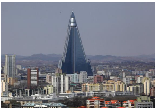
Figure 2: Ryugyong Hotel by Baikdoosan Architects, 2011 in North Korea.
