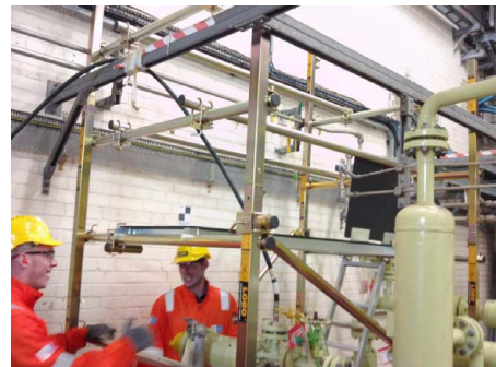
Figure 3: Tower 3: 1.8 × 2 × 4 m, Erected over K710 Flash Gas Skid.
