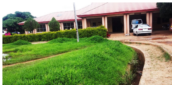
Figure 3: Plate III-Gwamna Awon general hospital Nasarawa road, Kaduna administrative block.
