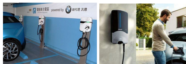
Figure 14: (a) Level Two Public Charging (b) Level Two Home Charging.
