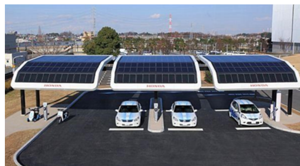
Figure 23: Solar Power Charging Infrastructures for EVs.
