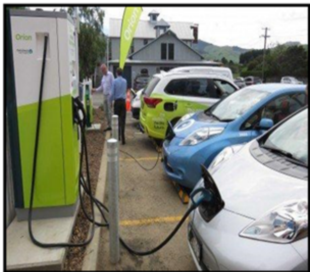
Figure 12b: Charging Point containing Several EVSEs.
