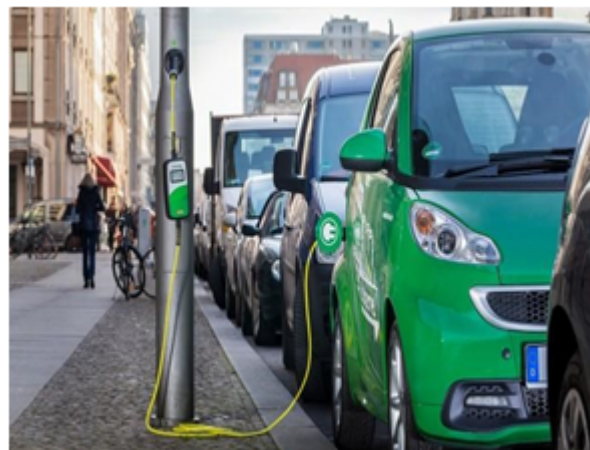
Figure 16a: Lamppost recharging of EV.
